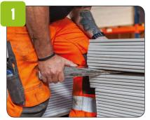
Insert a metal wedge in one corner to separate the required number of plates from the stack.
